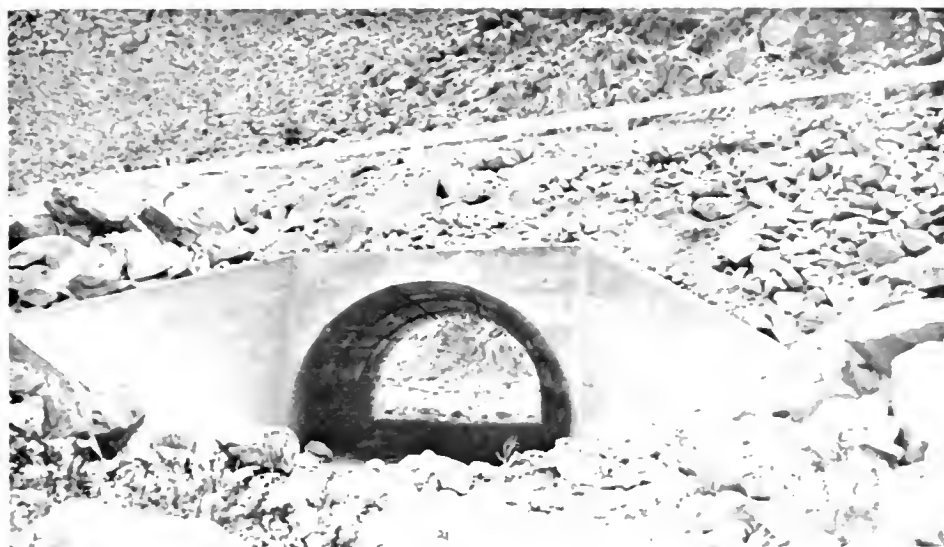
FIG. 54. Myers Creek culvert on State Highway in Imperial County, a flat arch under a low fill
